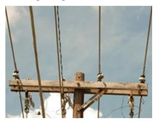
Outages caused by "tracking" can occur when dust accumulates on the insulators of utility poles and then combines with light moisture, usually caused by fog or drizzle. When there is a long dry spell, dust builds up on equipment. Light moisture combining with dust acts as a conductor, causing equipment to fail. It is possible that these outages result in a spark and pole or equipment catching fire. In such dry circumstances, it is beneficial to get a harder rain to wash dust away.
