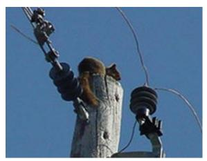
Squirrels, snakes and birds can come in contact with equipment such as transformers and fuses and cause equipment to momentarily fail or shut down completely. Many times, these critters are looking for a warm spot or food. Westar installs guards and protective fencing and uses various methods to help protect equipment.
